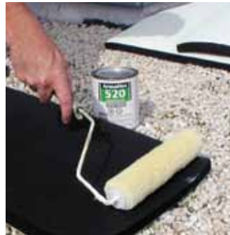
3. Roll thin coat of 520 Adhesive to insulation.
