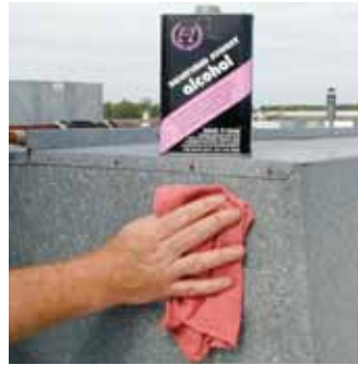
1. Always prepare surface by cleaning with denatured alcohol.
