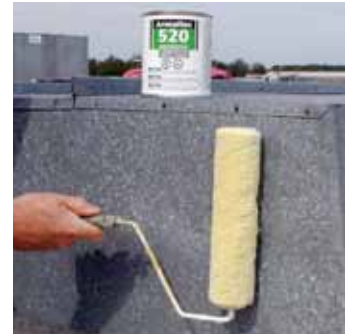
2. Apply thin, uniform coat of Armaflex 520 Adhesive.
