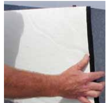
4. Position carefully and apply ArmaTuff. Contact adhesive bonds instantly.
